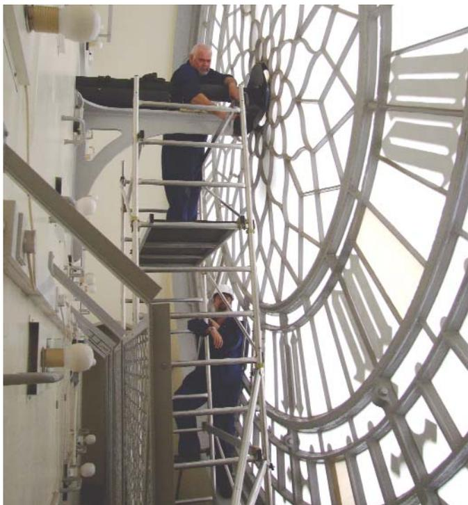
20. Scaffold behind dial to access the hour tube and minute arbor rollers.
